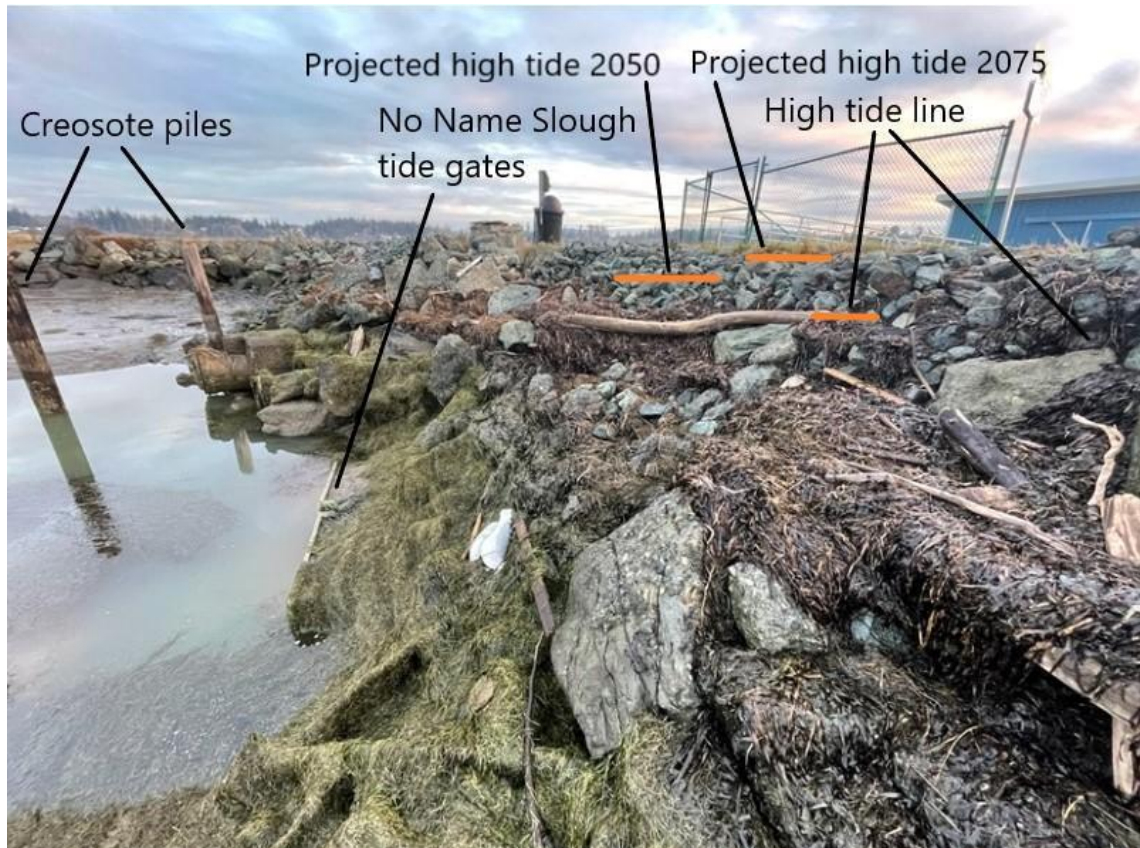
Figure 7. Padilla Bay side of No Name Slough with current and approximate future high tide elevations as projected using a 50% chance of occurrence from CIG models using high greenhouse gas scenarios (CIG 2024).
