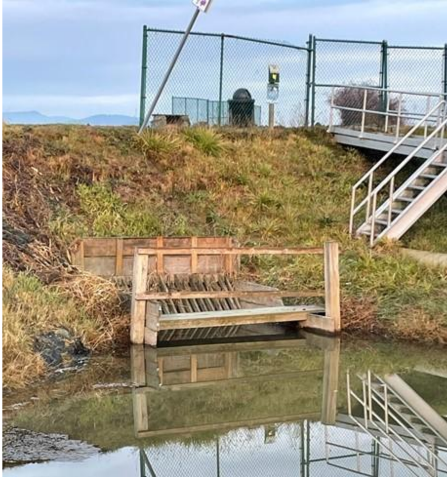
Figure 3. Trash Rack (approximately 12 feet wide) on the Slough side of the No Name Slough tidegate. The trash rack is proposed for removal. Photo credit: Jenna Friebel.
