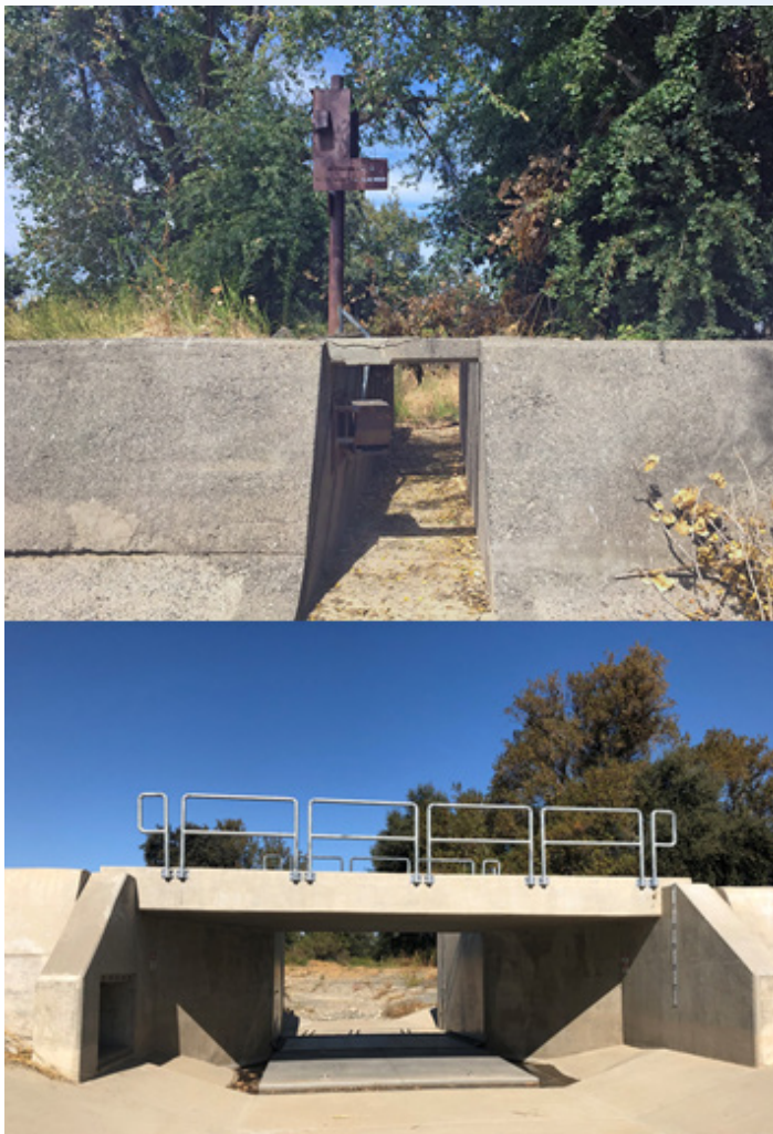
Fremont Weir fish ladder in 1965 (top) and 2018 (bottom). The new fish ladder provides much improved passage for adult winter-run Chinook salmon to return to the Sacramento River from the Yolo Bypass. Credit: U.S. Bureau of Reclamation
