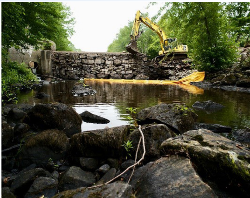
The removal of the Coopers Mill Dam on the Sheepscot River in Maine. Credit: Tim Swan
