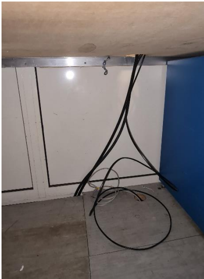
Figure 44. Main &amp; spare deck cables under PAM desk.
