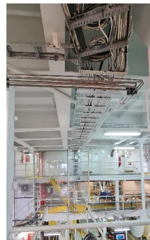
Figure 47. Aft wall of server room with cable tray.
