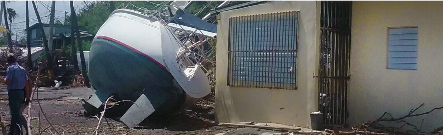
Damaged facilities in Punta Santiago, Humacao (top); Damaged facilities in Playuela, Aguadilla (middle); Sailboat washed ashore in Sardinera, Fajardo (bottom). Photos: Puerto Rico's Department of Natural and Environmental Resources/Luis Aníbal Padilla-Rivera
