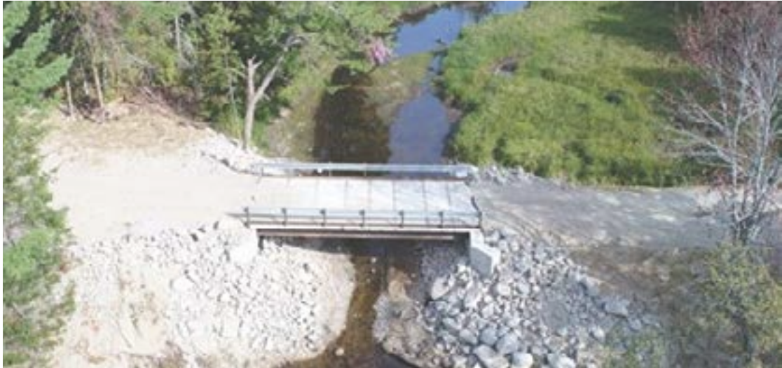
Photo Credit: Project SHARE culvert replacement
