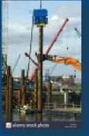
Today, we will be walking through two examples, starting with an impact pile driving example (36" steel pipe piles, 3 piles per day, 1000 strikes/pile, with a bubble curtain).
