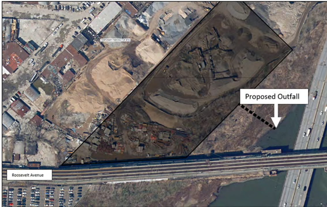
Figure 3 – Aerial View of Temporary Stormwater Outfall at the MTA/Tully Site
