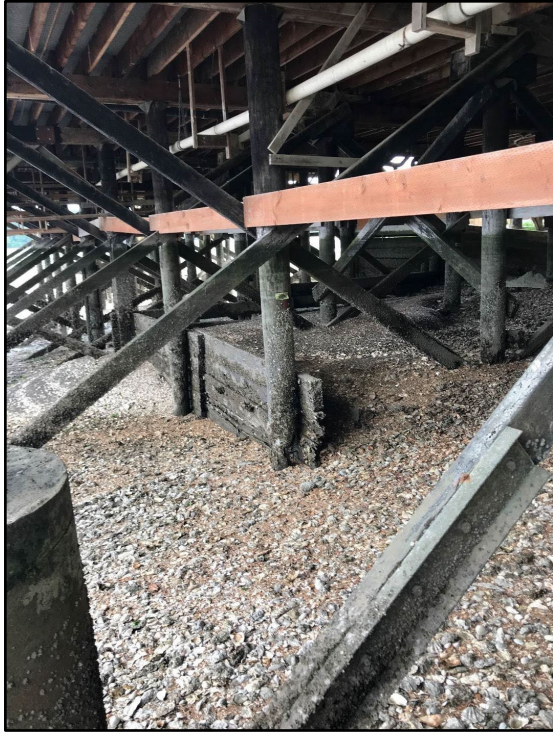
Figure 19. Removal Credits for Non-Functional Shoreline Armoring that is not in good condition. Removal credits do not apply for horizontal pile stabilizer as there is no functioning bulkhead effect (like sediment retention behind the bulkhead or elimination of water exchange).
