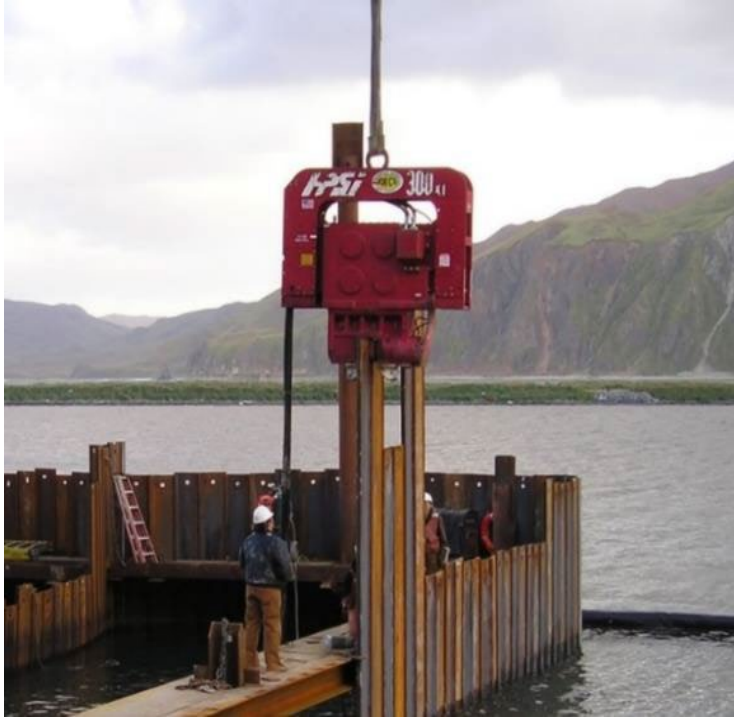
Figure 1-4. Installing sheet piles with a vibratory hammer.
