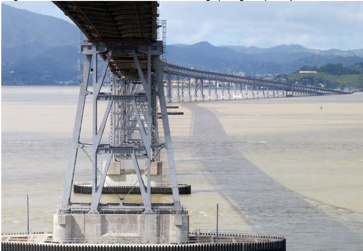
Figure 1-4. View of the Richmond-San Rafael Bridge (facing west) from pier 48
