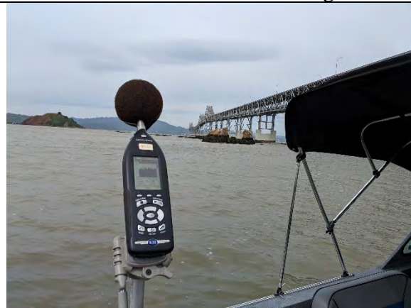
ST-2: ~195 feet from the edge of the Richmond-San Rafael Bridge
