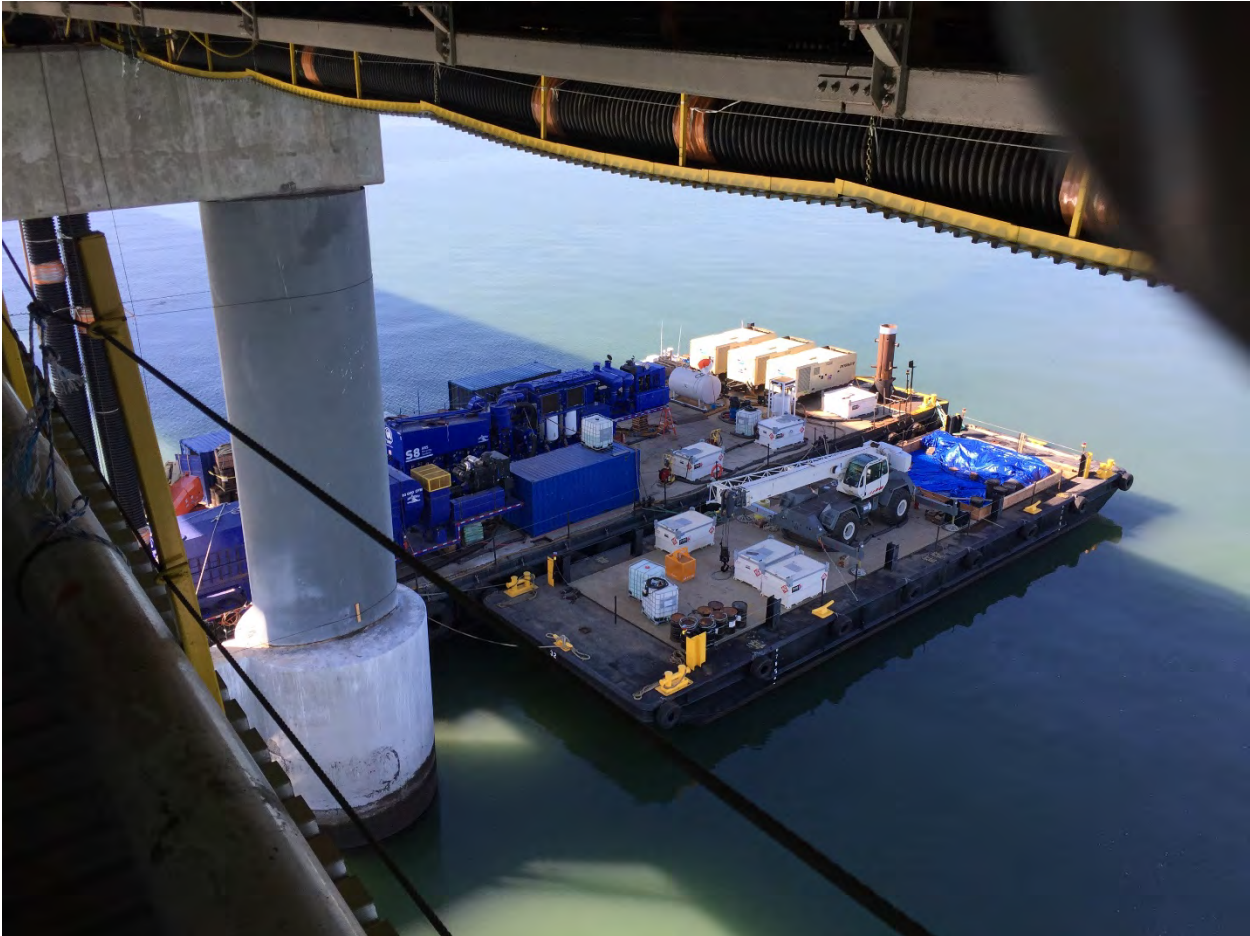
Figure 5-1. Photograph of Barge to be Used in Construction
