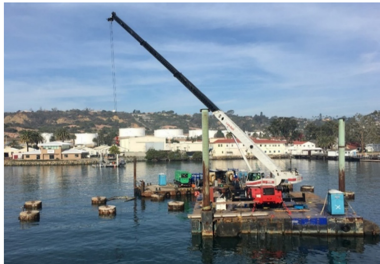
Figure 30. Removal of 84-inch Caissons using a Mactech DWS-102i 102-inch Inline Hydraulic Feed System Diamond Wire Saw.
