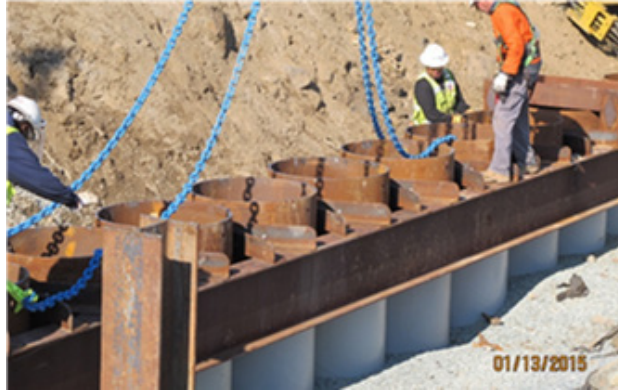
Figure 16. Configuration of 36-inch Steel Abutment Piles.
