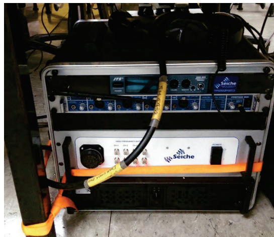
Figure F-4: DPU and deck cable in the main lab.
