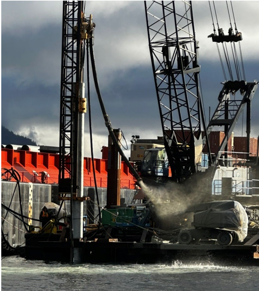
Figure 7. Drill 30-in. diameter socket at berthing dolphin S4.
