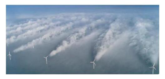
This is a photograph of massive cloud trails caused by blade rotation of the turbine blades at the Horns Rev Wind Turbine Power Plant in Denmark.
