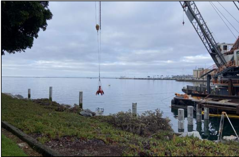
Dredging (in-water work) at the Project Site on August 29, 2022. Facing southwest.
