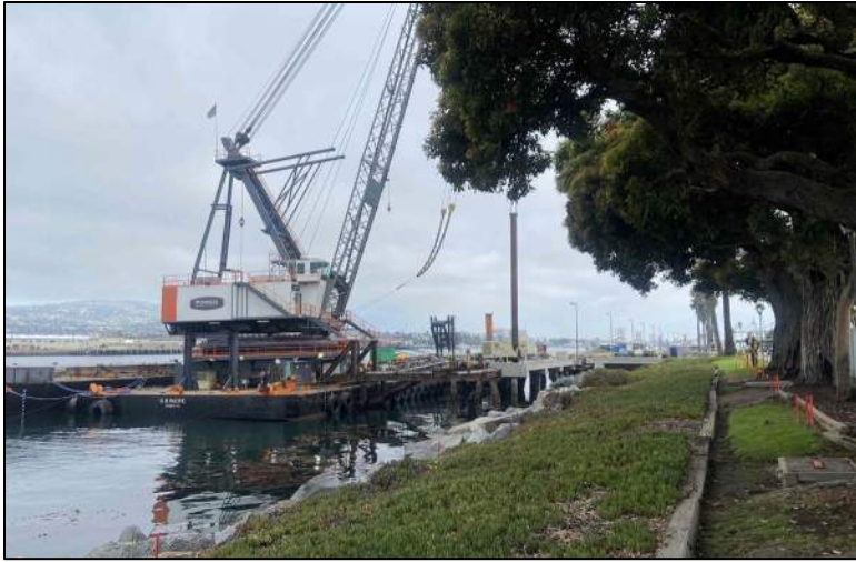
Pile drive testing at the Project Site on June 29, 2022. Facing northwest.
