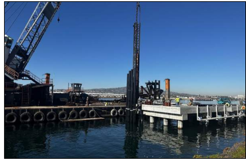
FRP piles installed at the Project Site on January 25, 2023. Facing west.
