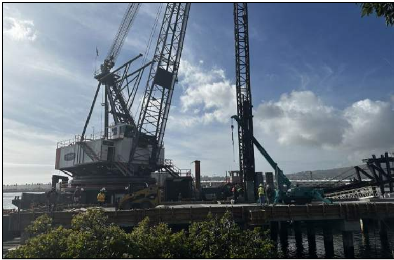
Pile driving at the Project Site on January 11, 2023. Facing west.
