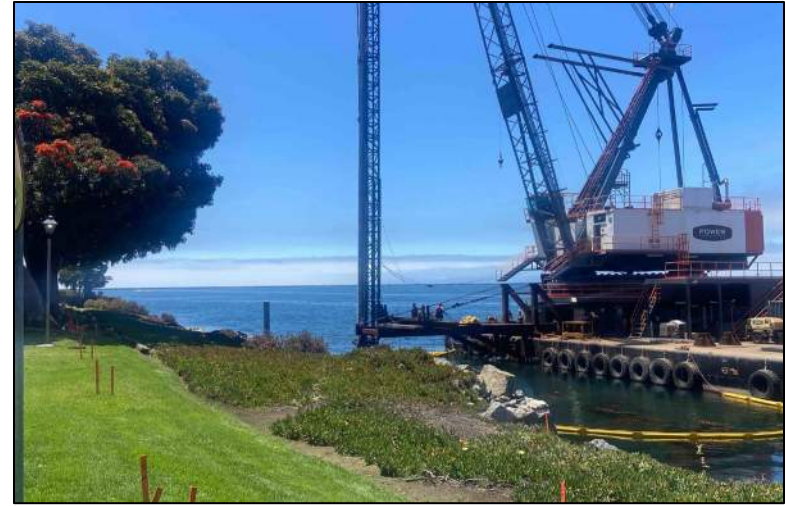
Pile drive testing at the Project Site on July 6, 2022. Facing south.
