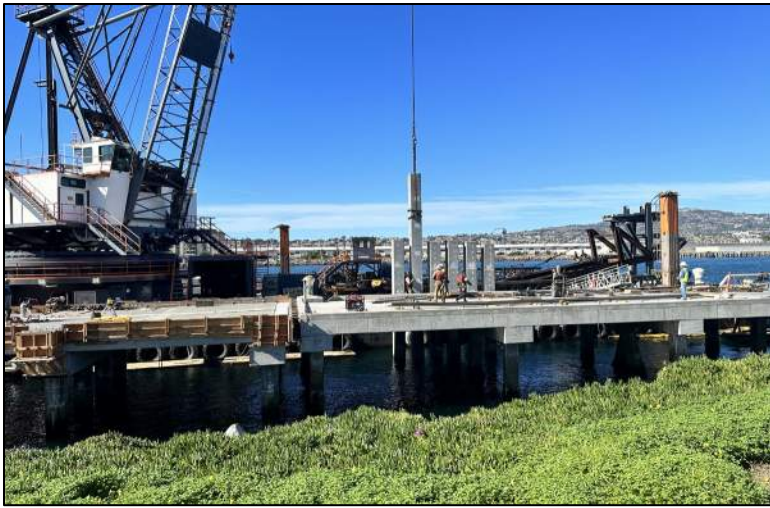
Fender pile pulling at the Project Site on November 3, 2022. Facing west.
