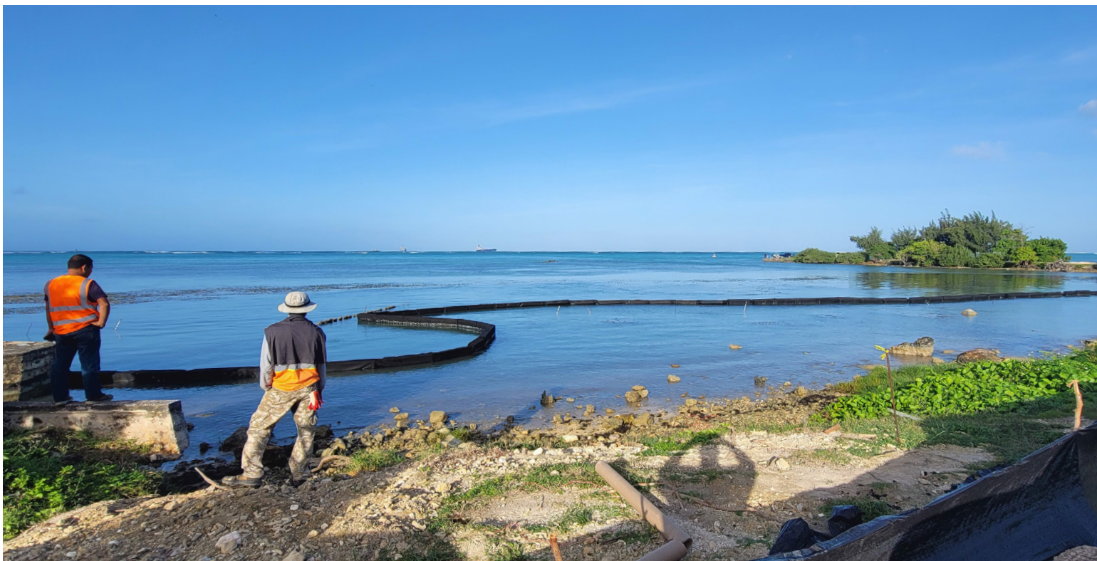
The CNMI DLNR installed water quality boundaries, shown in black, to protect the environment during an improvement project at the Garapan Fishing Base in Saipan. The project will build 12 steel pavilion structures, or palapala, to support local fish vendors. Credit: WPFMC
