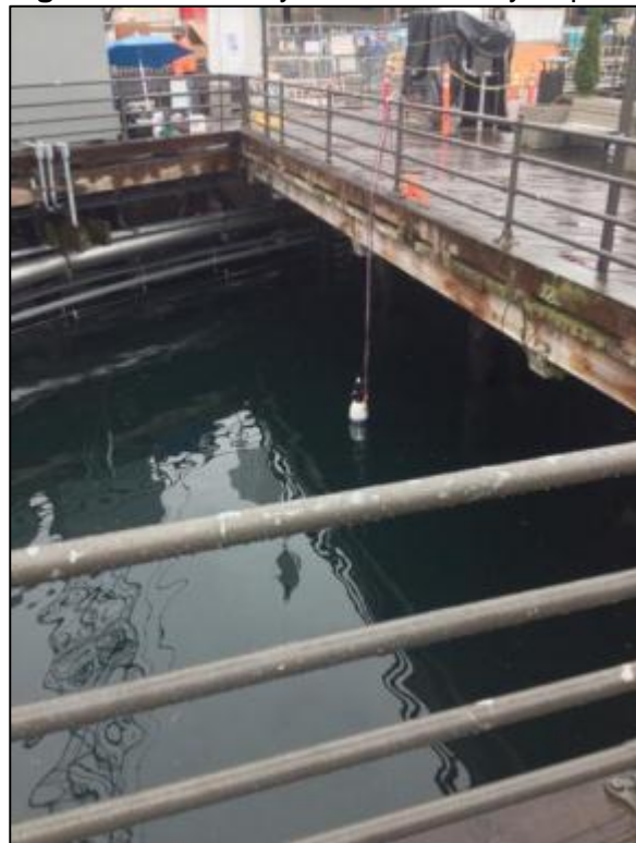
Figure 8.3 Vibratory Sheet Pile 1 Hydrophone
