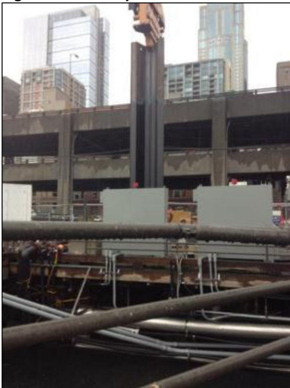
Figure 8.2 Vibratory Sheet Pile 1
