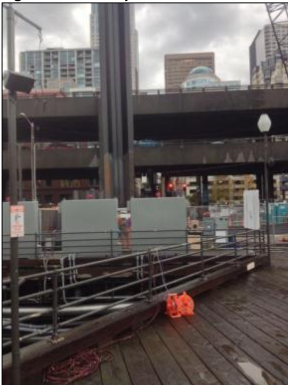
Figure 8.9 Vibratory Sheet Pile 2
