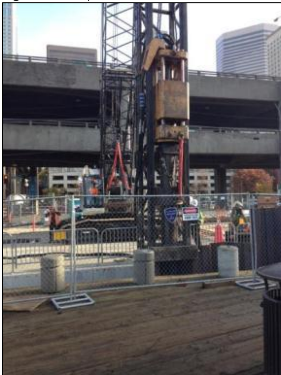
Figure 9.10 Impact Sheet Pile 2
