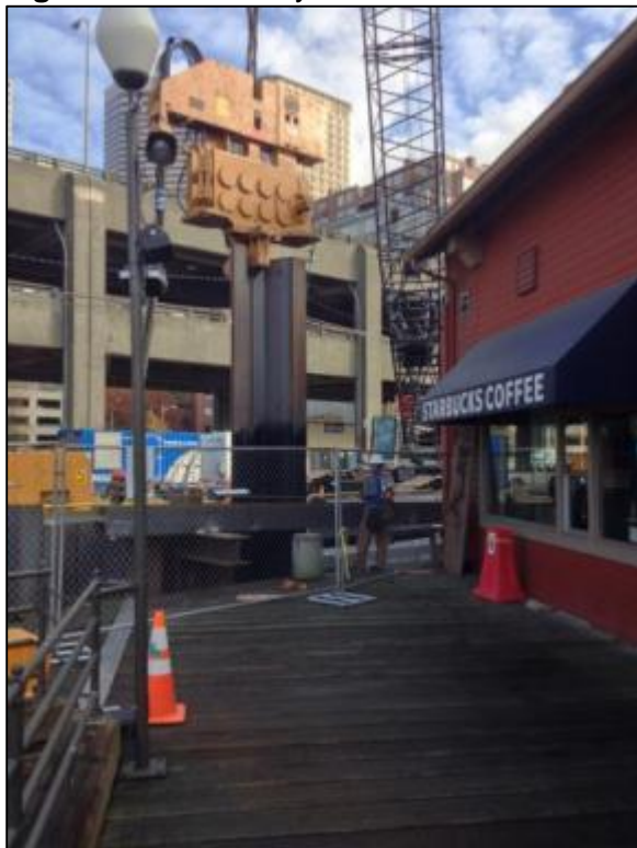
Figure 8.30 Vibratory Sheet Pile 5
