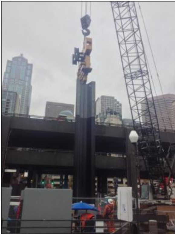
Figure 8.23 Vibratory Sheet Pile 4
