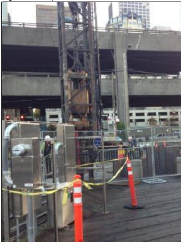
Figure 9.2 Impact Sheet Pile 1
