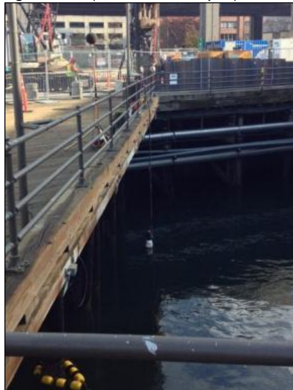
Figure 9.19 Impact Sheet Pile 3 Hydrophone
