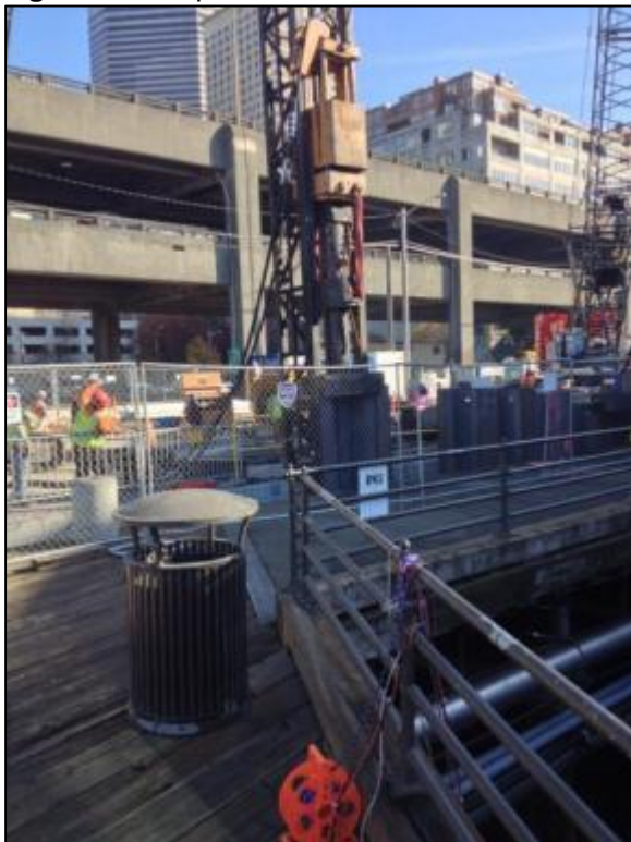
Figure 9.34 Impact Sheet Pile 5
