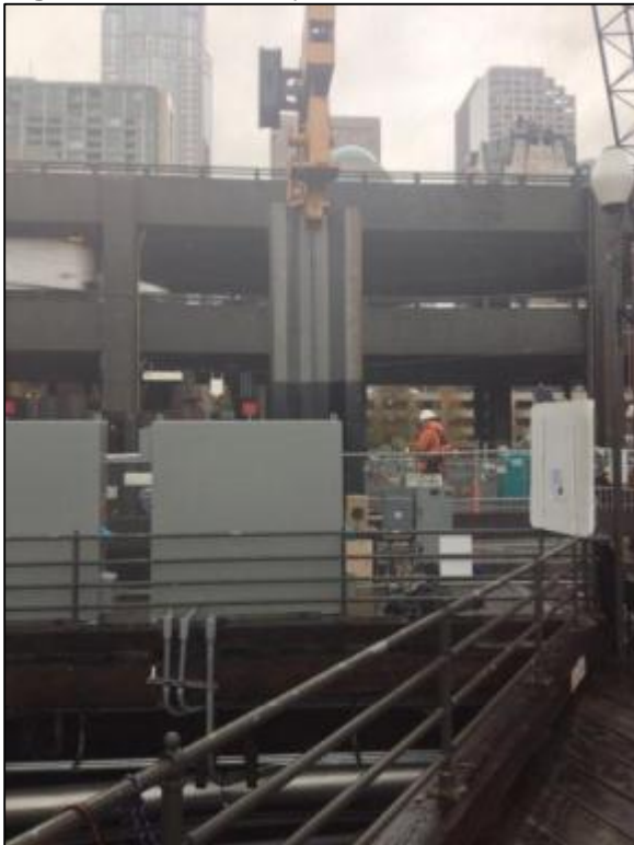
Figure 8.16 Vibratory Sheet Pile 3
