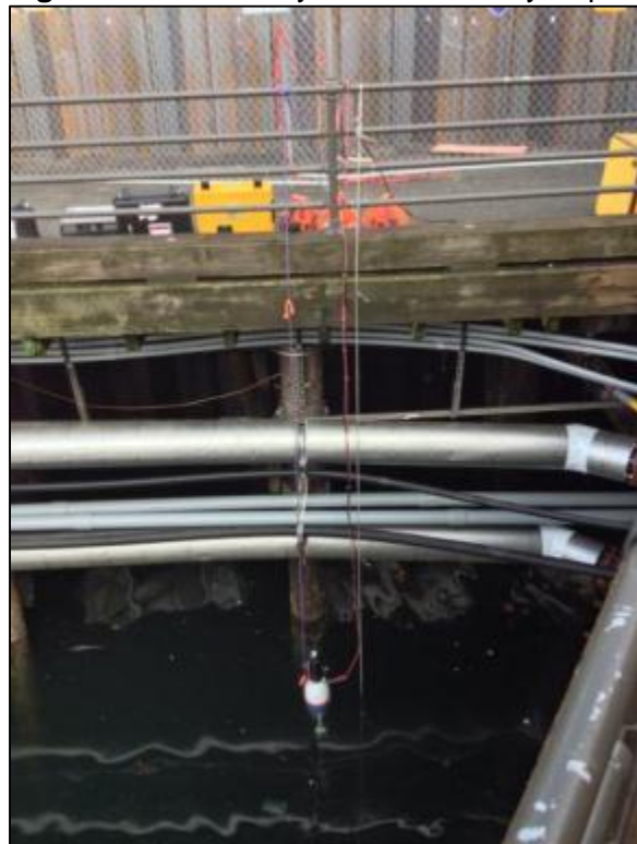
Figure 8.31 Vibratory Sheet Pile 5 Hydrophone
