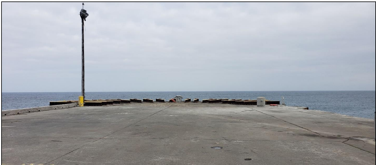
Figure 1-7. View of Pier Deck
