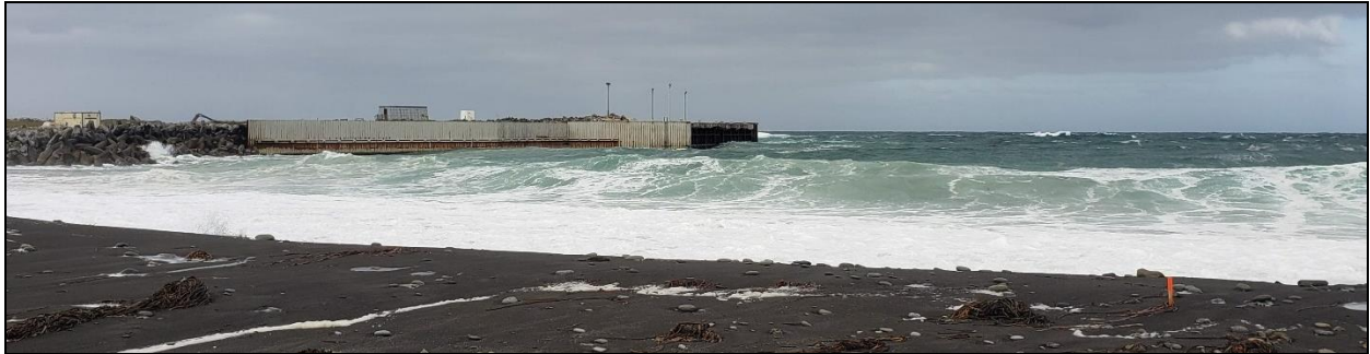
Figure 1-2. View of Eastern Berth of Pier from Alcan Beach
