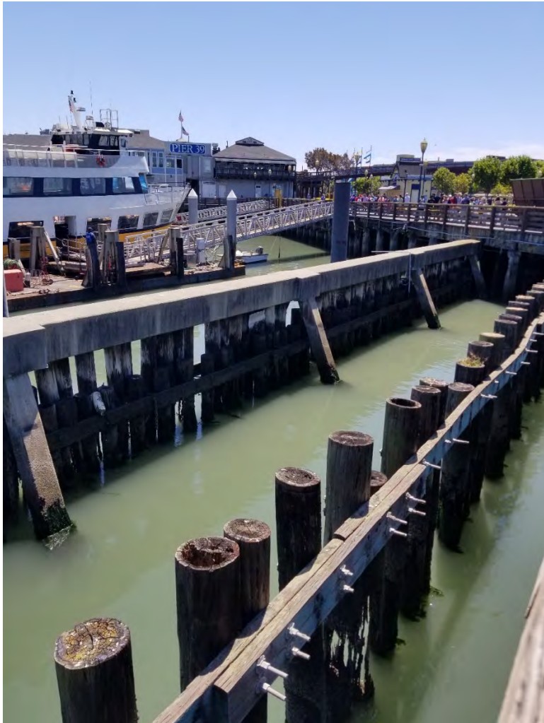
Photograph 4: Taken between Piers 39 West Basin and 41 ½ looking south.
