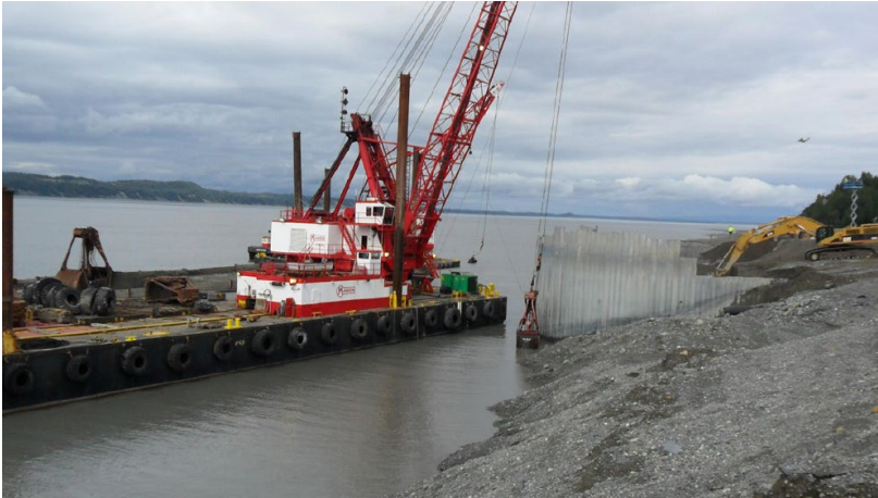
Figure 1-9. Manson Derrick Barge VIKING Dredging near OSCP™ Bulkhead (Source: Manson)
