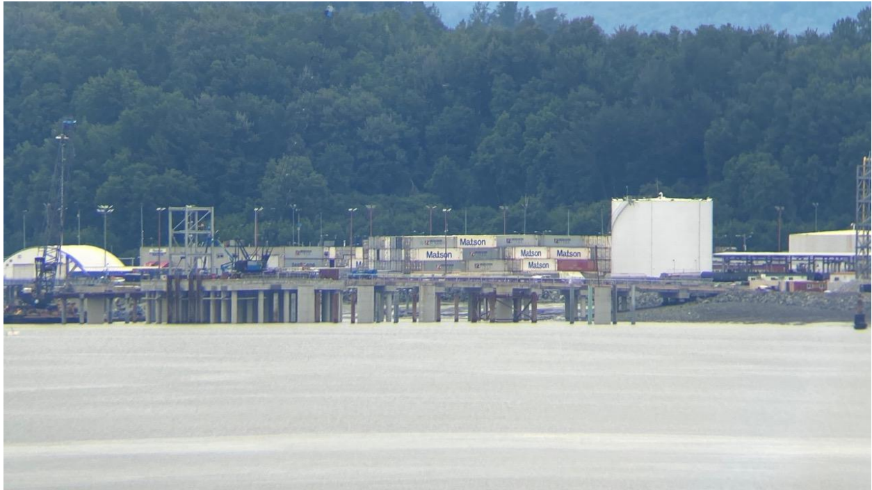
POA PCT Dock Construction
