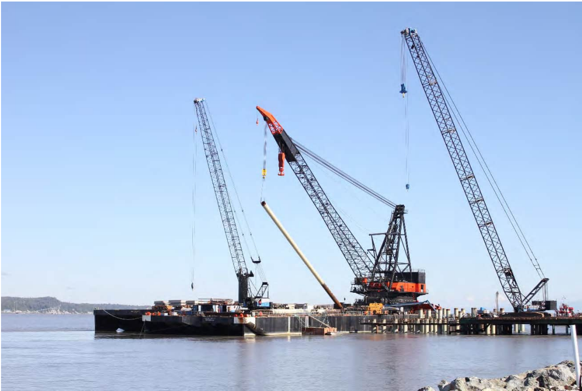
Photo 2. View of PCT construction from PCT PSO Station
