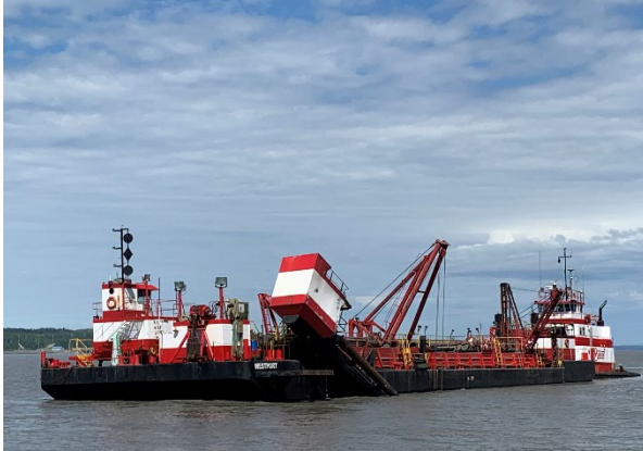
(a) Dredge disposal offshore of PCT construction area
