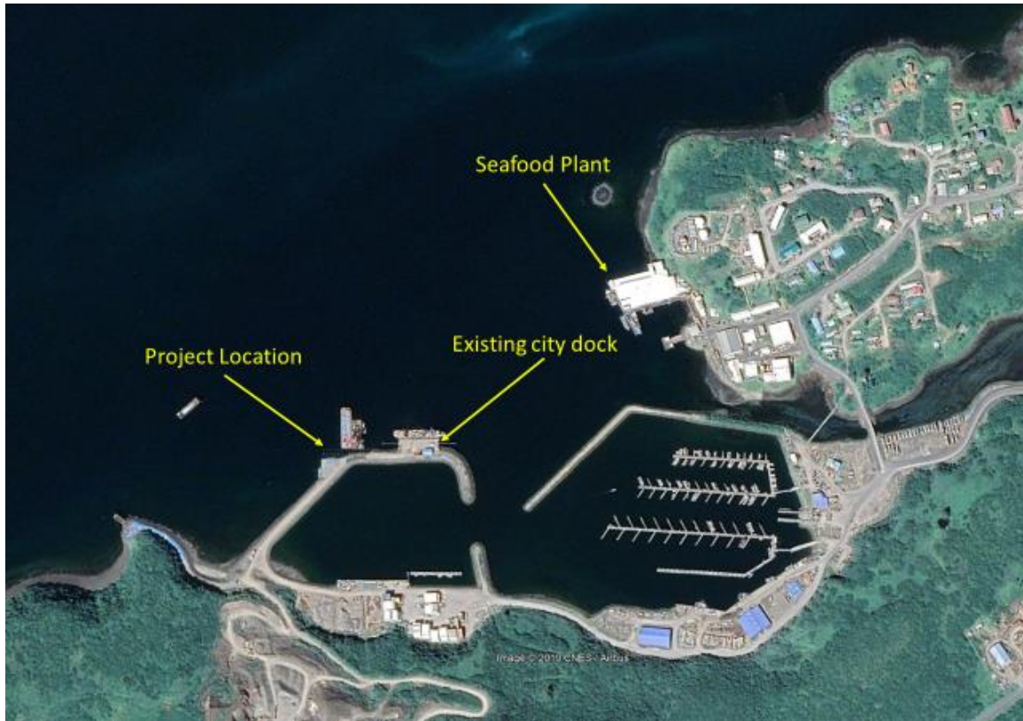
Figure 1. Project location within Sand Point, AK. This image shows the project under construction.
