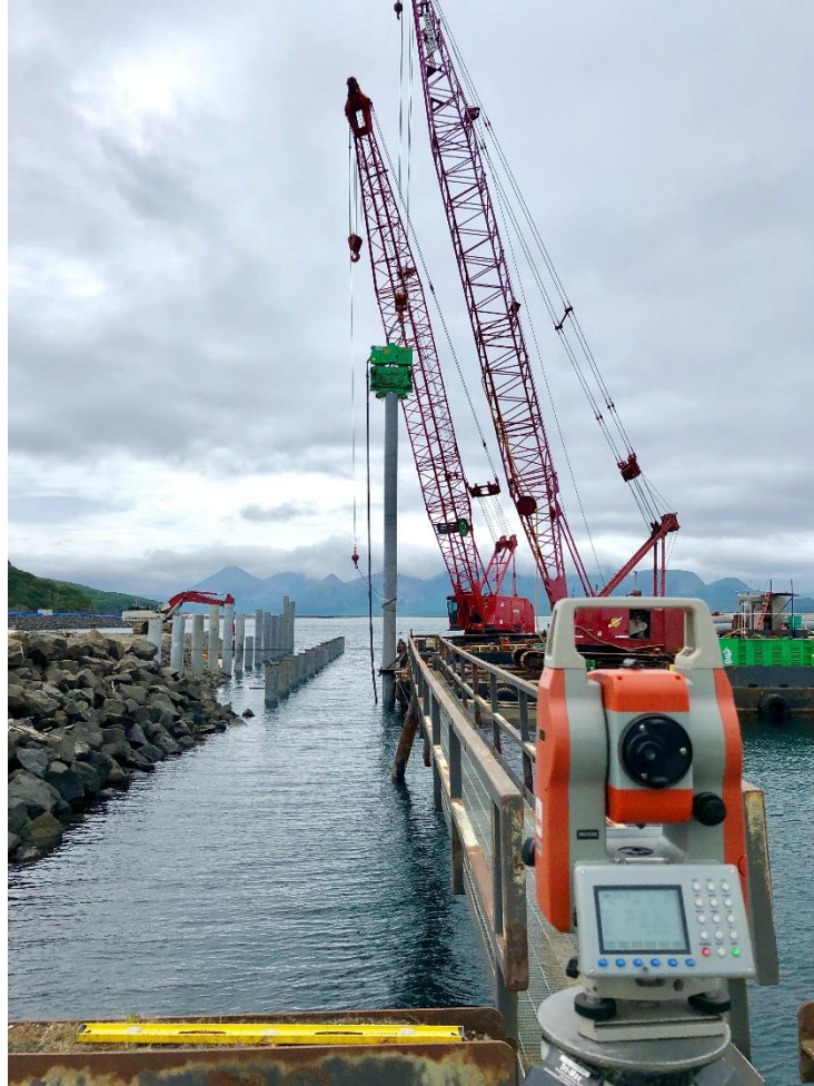
Figure 2 – Vibratory pile installation
