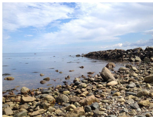
Cobble/boulder pavement (not including groin) Credit: K. Shaw
