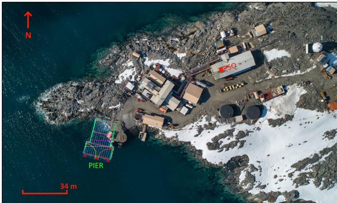
Figure 6. Aerial view showing the locations of the pier site and PSO observation shelter during in-water construction activities at Palmer Station, 23 January–14 June 2022. Note: PSOs monitored from the new pier and science office during anode installation.
