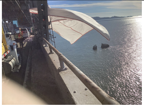
Photo 4: API attaching tarp at Pier 55 (11/11/2023)
