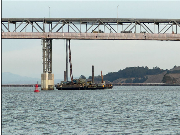
Photo 3: Scaffolding and containment between Piers 51 and 52, barge stationed during sandblasting (10/31/2023)
