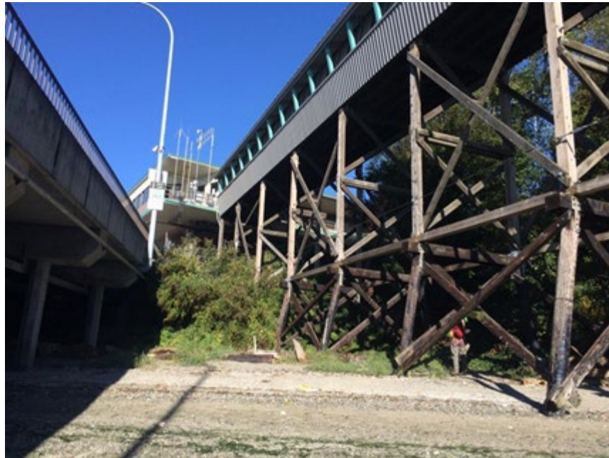
Figure 3-2 Existing Timber Walkway to be Removed
