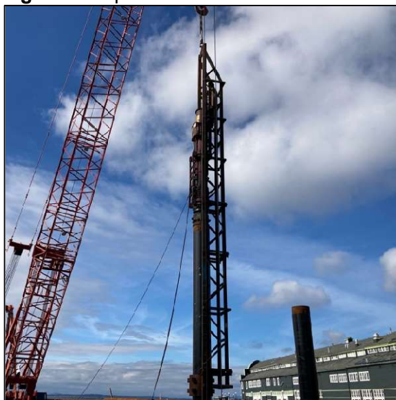
Figure 3. Impact Pile Driver
