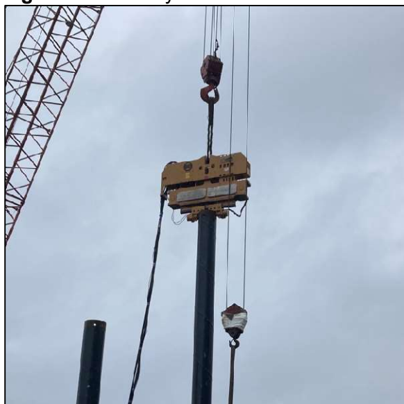
Figure 2. Vibratory Pile Driver
