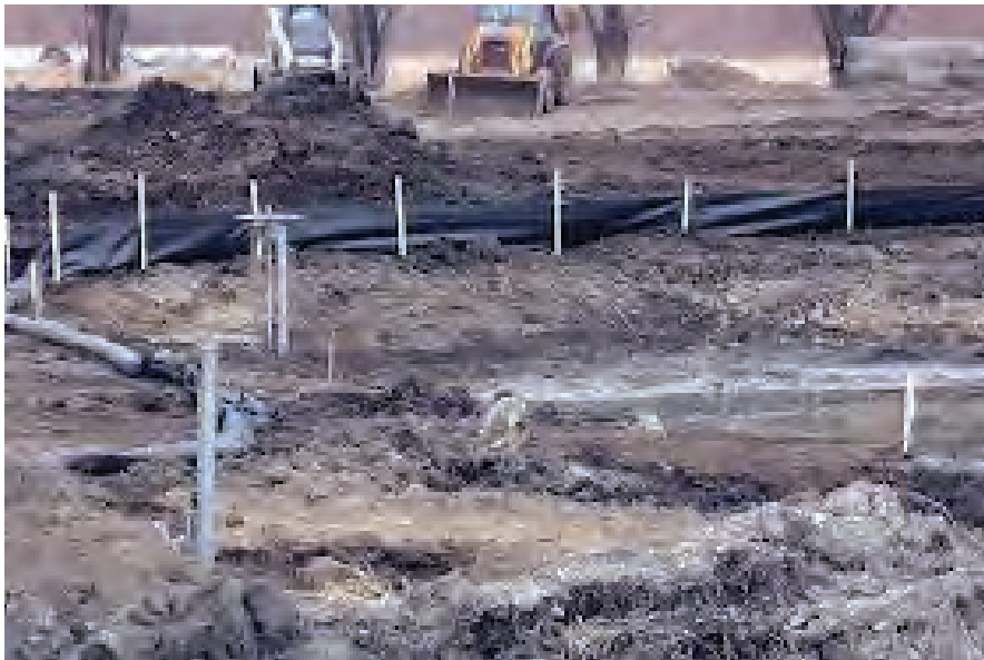
Photo C. Silt Fencing around a channel
