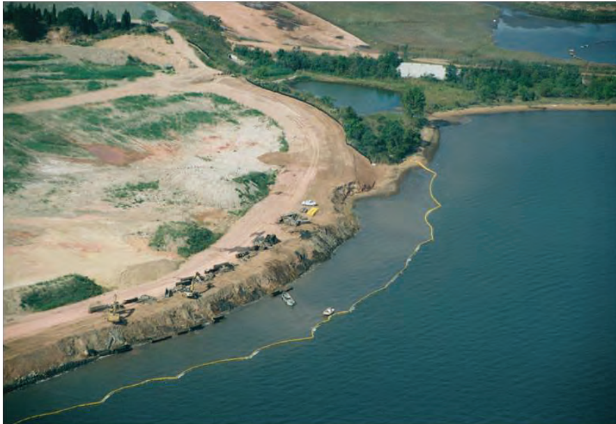
Photo A. Turbidity control with containment fencing
